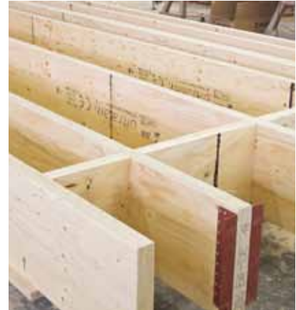
Pre-assembled box girders for roof construction.
